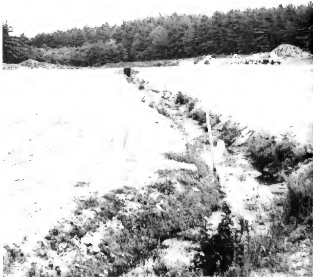
Presently: work in progress
